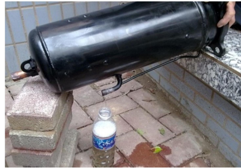
Figure 4-4.10: Draining oil from a compressor
